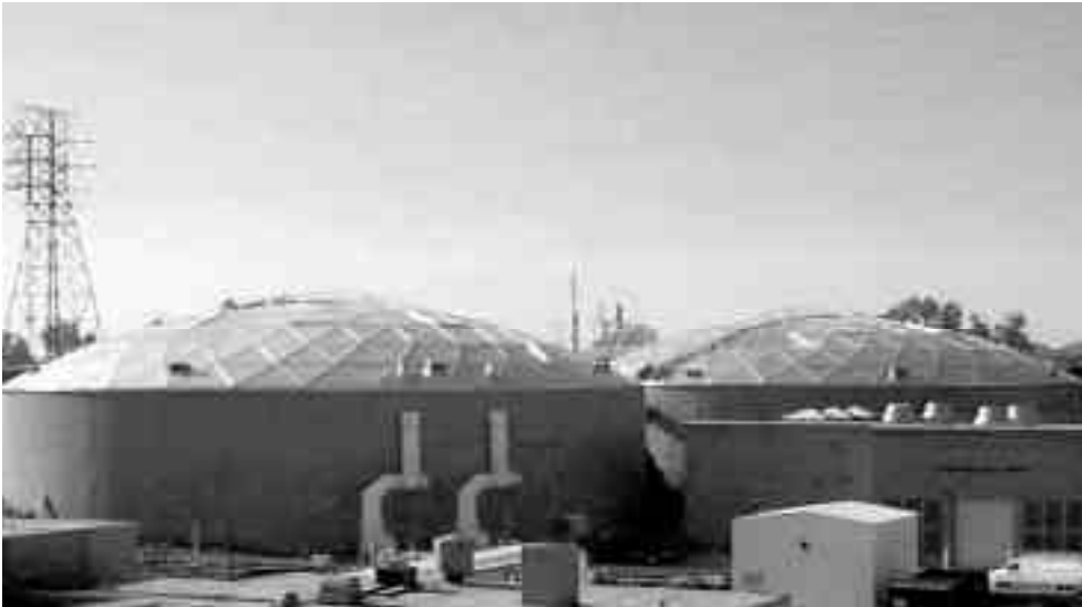
Installed in 1994, bioroughing towers pretreat high-strength wastewater at the Morris Forman facility by using bacteria to break down solids. To reduce the potential for odors, aluminum dome covers were added to the towers in 1999.
