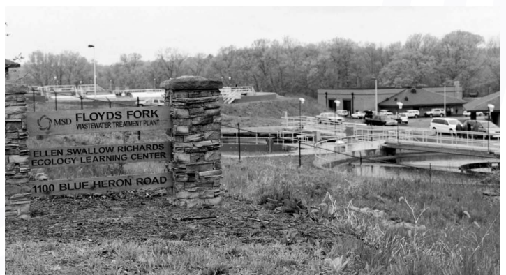
MSD's Floyds Fork Wastewater Treatment Plant was recognized as the utility Project of the Year by the Kentucky Chapter of the American Public Works Association.
