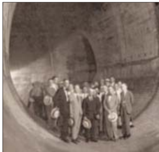
Built in the early 1930s, the Southwest Outfall is one of the oldest and largest underground structures in MSD's system.
