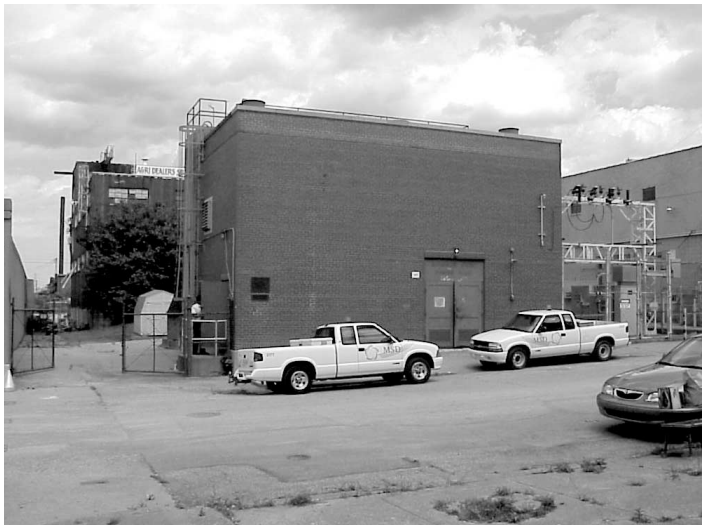
The 50-year-old Buchanan Street Pump Station is critical to MSD's sewer and flood protection systems.
