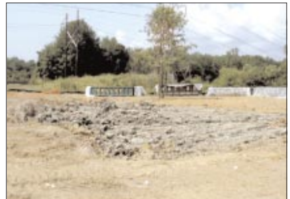
Wastewater once treated at the Confederate Acres plant has been diverted to a plant with greater capacity, saving cost and reducing the risk of pollution.
