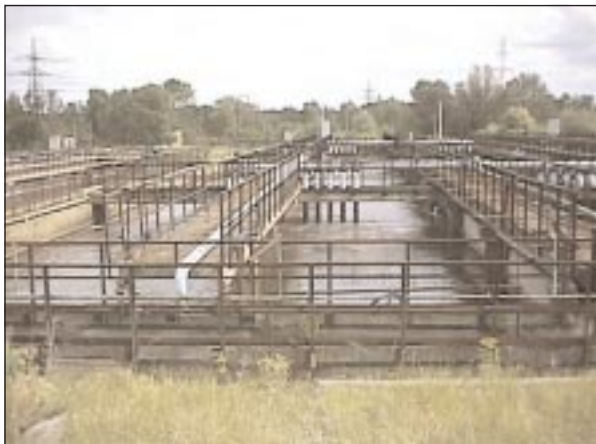
One wastewater treatment plant, operated by a chemical manufacturer, serves most of Rubizhne's 70,000 citizens.
