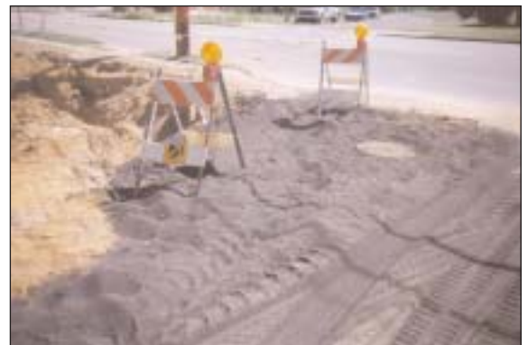
Black sand from electric power plants works like sand on a construction site but is cheaper to haul.
