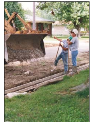
Project DRI at work
