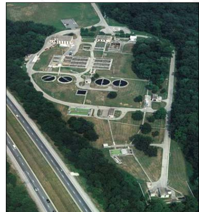
Expansion of the Hite Creek plant will allow the treatment of an additional 1.6 million gallons of wastewater per day.
