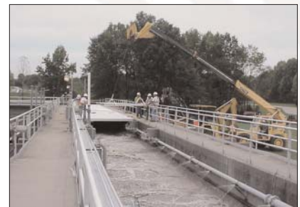
Channel covers will enclose many of the wastewater treatment areas to capture odors.
