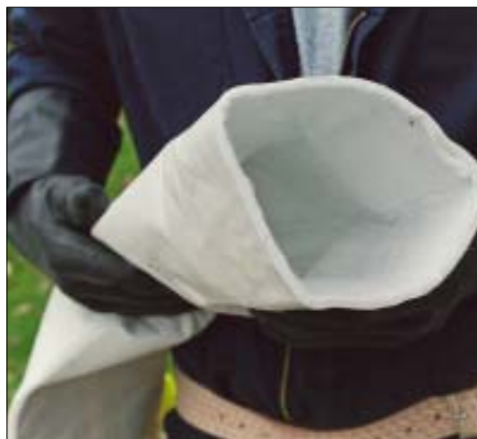
The PVC-based liner is prepared above ground and injected by air-pressure to trouble spots in main sewer lines and property service connections, eliminating the need for excavation.
