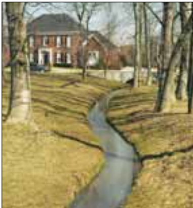
Drainage facilities like this will be maintained by MSD under an agreement with the City of Prospect to provide drainage services.
