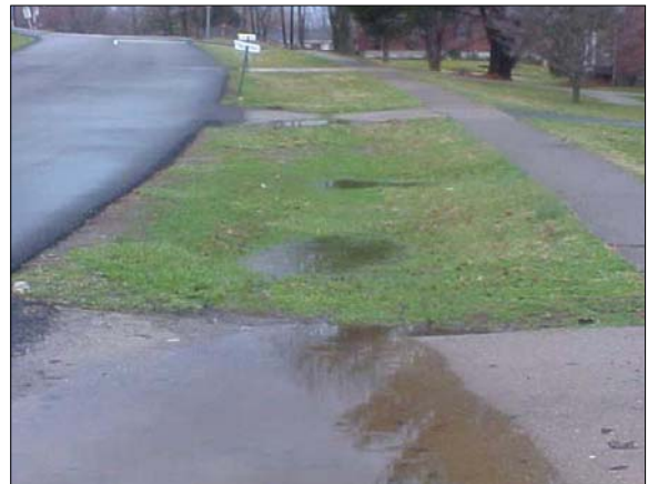
Adequate drainage facilities don't exist in many suburban Louisville Metro neighborhoods, like Woodland Hills south of Shelbyville Road.
