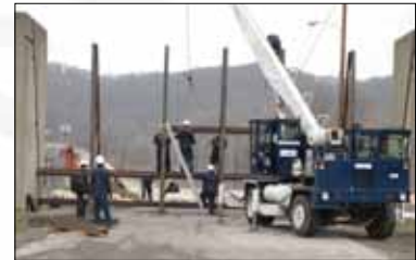
Crews install a flood protection street closure at Riverport.
