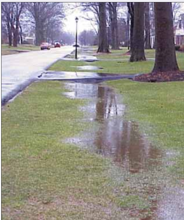
Project DRI continues to work in neighborhoods across Louisville Metro, like this one near St. Matthews, to upgrade existing drainage facilities and build new ones.
