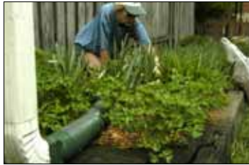
Stormwater from a downspout is directed to a rain garden for thriving plants and to reduce the stormwater burden on combined sewers.
