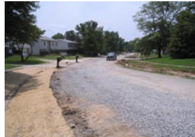
A sewer rehabilitation project along Running Fox Circle has corrected low spots in the sewer line which have caused repeated backups for 13 of 30 area properties in the past five years.
