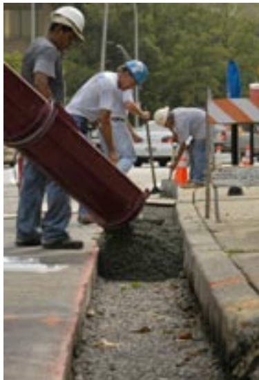
Above: Porous concrete is installed in a two-foot strip along the curb of Liberty Street to catch stormwater runoff before it enters the drainage system.
