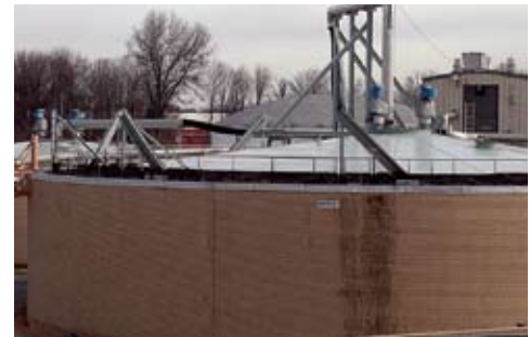
Digester 2 at the Morris Forman Water Quality Treatment Center will be cleaned to maintain efficiency and preserve its original design volume.
