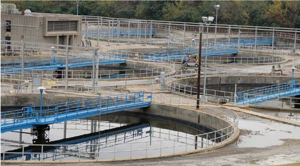
National Water Services (NWS) will replace two failed pumps and add another well and pump to stabilize groundwater for the clarifiers at the Morris Forman Wastewater Treatment Plant.
