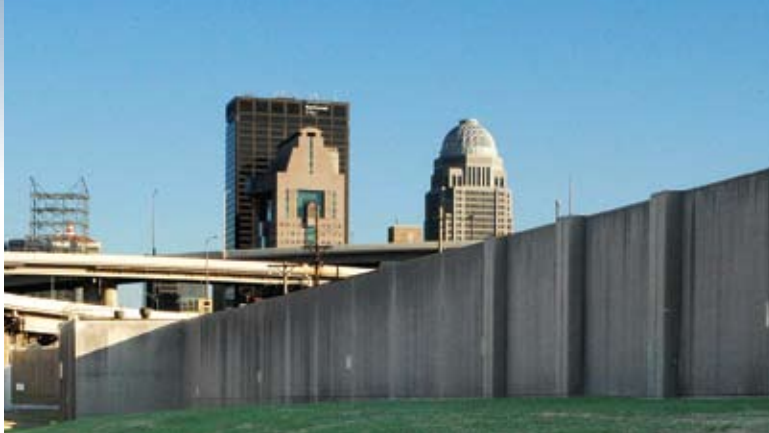
A portion of the Flood Protection System in downtown Louisville.
