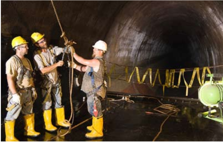
John Rice, Rob Jacobs and Mike Rice (MAC Construction) install an inflatable rubber dam (or gate) inside the Southwestern Outfall as normal dry-weather flow passes through the conduit beneath them.
